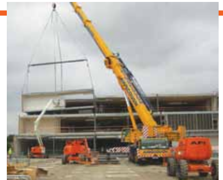
AFI machines working on the construction of the catering village.
